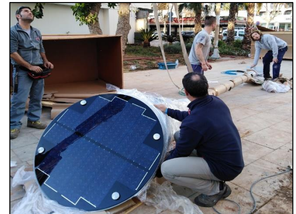
Installation works of TULIP SSL in Hotel Meliá
